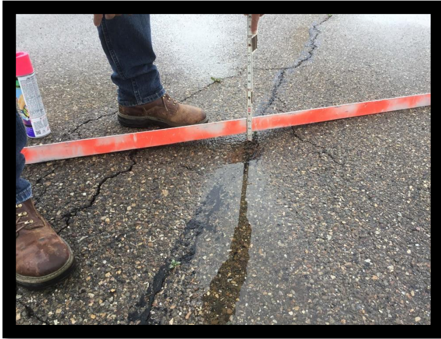
TERMINAL APRON, SECTION 2, SAMPLE UNIT 18 – Distress Type: Rutting
