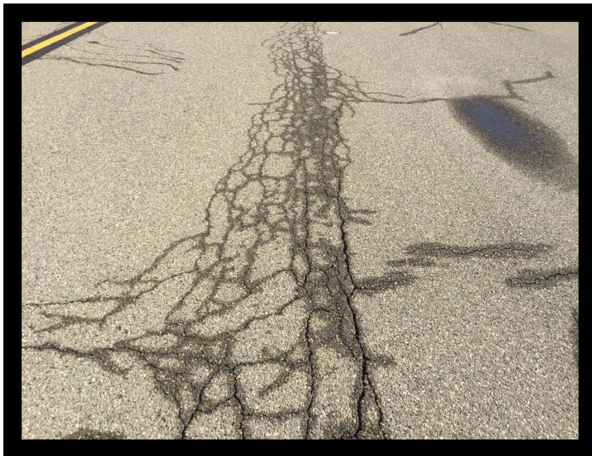
TAXIWAY T, SAMPLE UNIT 2 – Distress Type: Alligator Cracking
