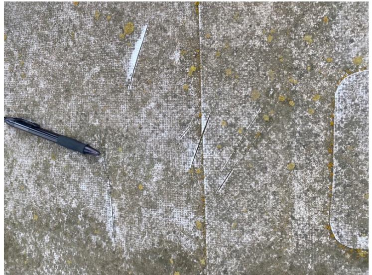
Cuts in membrane; leak location
