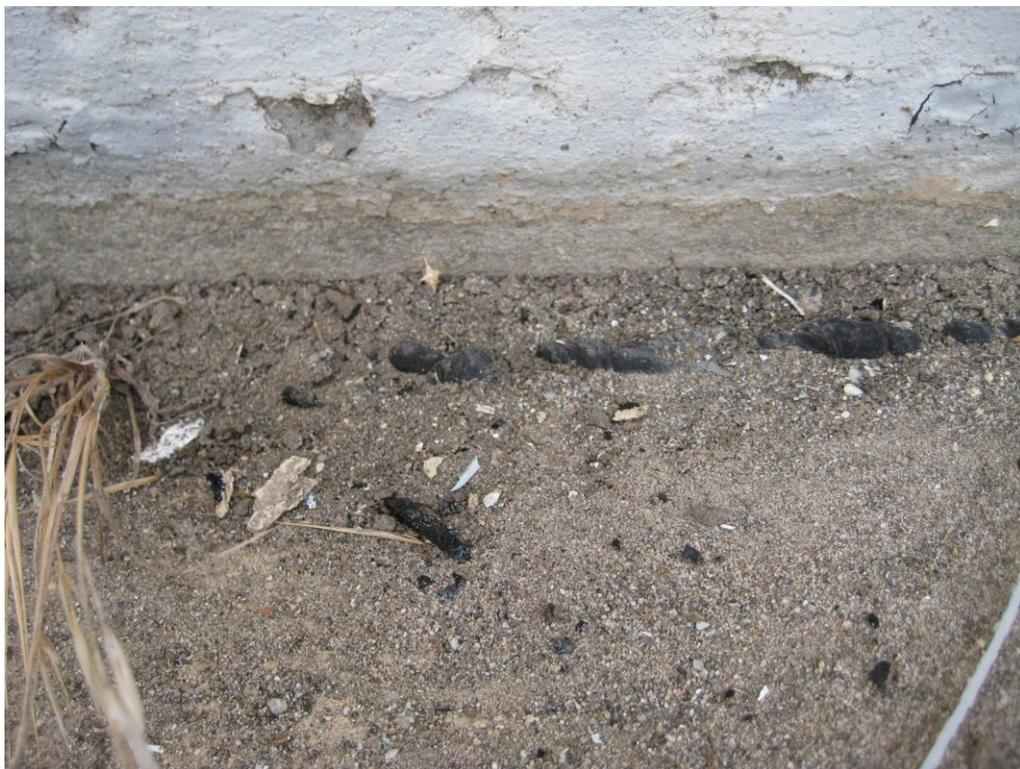
Photo depicting soil accumulation at drip line on east elevation on top of caulk material
