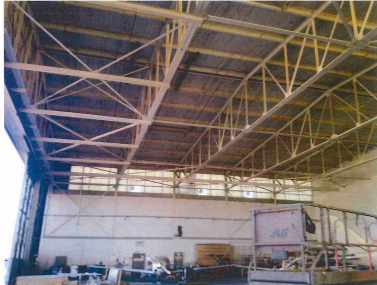
bottom chords around the perimeter of the hangar bay and roof truss bottom chord bracing to prevent buckling when the roof experiences uplift due to wind forces. The office spaces feature columns at the exterior walls that align with the main hangar columns.
