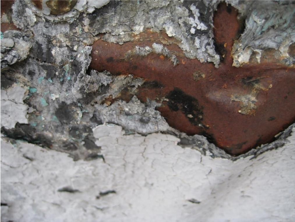
Degradation to Layered Coating and Substrate
