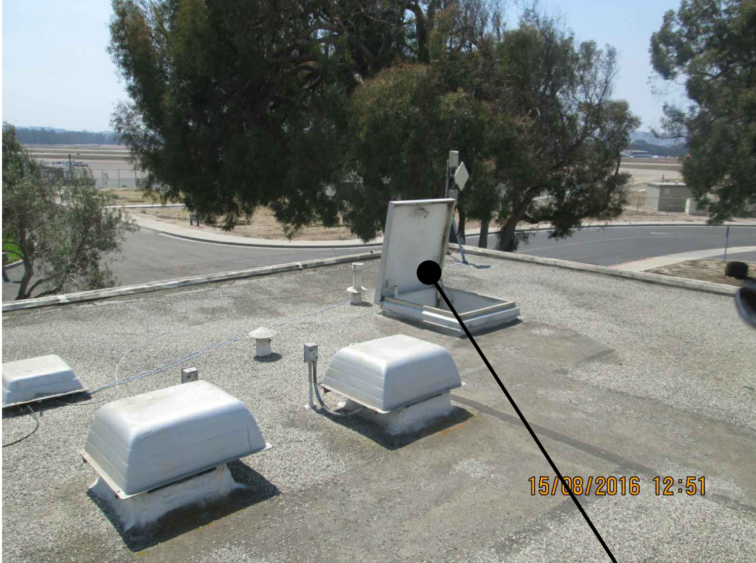
(N) HATCH & UP LADDER POST PHOTO
